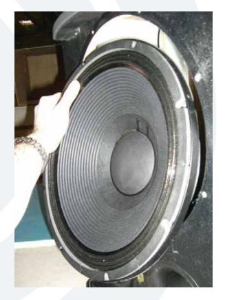
Carefully begin to remove the woofer. This woofer has a tendency to want to pop out, so please be sure to hold the woofer in place with your free hand while removing the screws with the other
